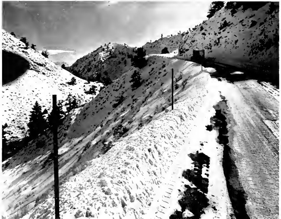
This section of Sherwin Grade north of the summit will be modernized to eliminate bad ascent and curves
